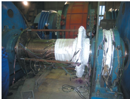
Fig. 6. Area around place of welding was isolated and then heated up with electric heating unit and heating mats. Heating speed was about 25^{\circ}\text{C/h} [1]
